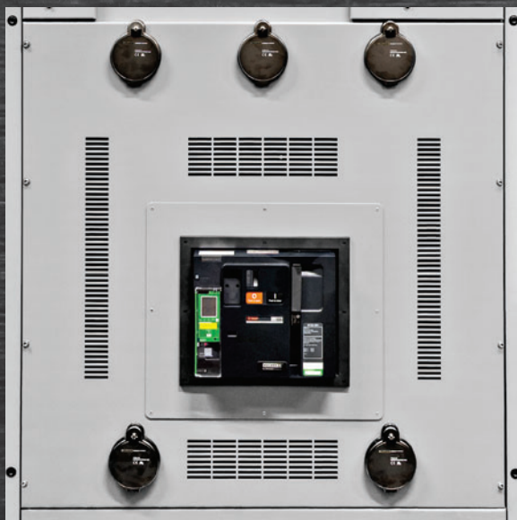
RETROFITTED SWITCHBOARD
